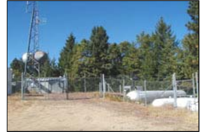
South Hoadley Peak communications relay facility.
