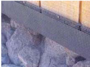
Cover openings with 1/8" metal screen to block fire brands and embers from collecting under the home or deck.
