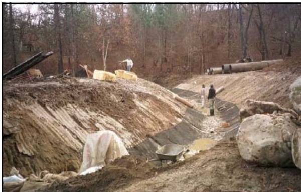
Lowden Fire Drainage Improvement on Landowner's Previous Home Site
