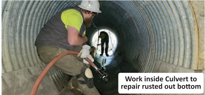
1506 mm 0.95 First section of road removed, channel armored and culvert bottom repaired October 2024
