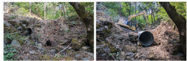
Hobo Gulch Road Culvert Upgrade (Old Culverts visible in the Upper Left Image) August 2024
