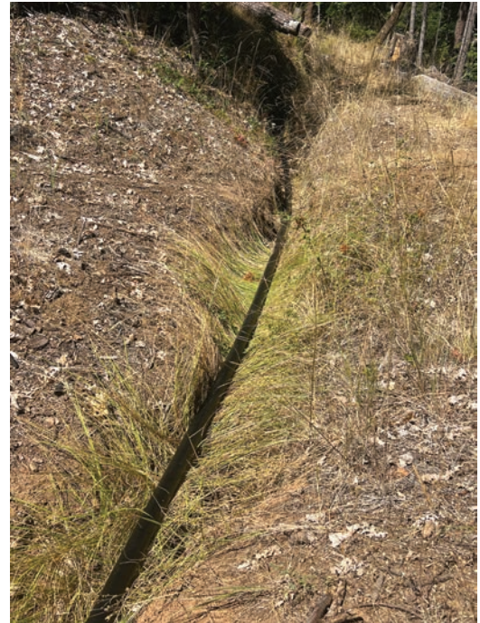
Plastic pipe installed in the ditch
