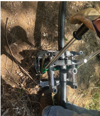
In this series of photos Boyd Butler and Jesse Brookings set the tee into clamp to fuse to the next section of pipe. They use a metal paddle run by the generator to heat the plastic on both sides and then clamp it together when hot to fuse the seams together
