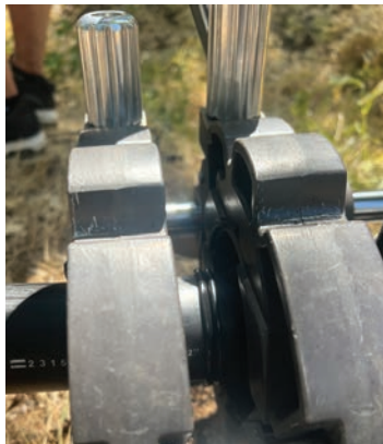
In this series of photos Boyd Butler and Jesse Brookings set the tee into clamp to fuse to the next section of pipe. They use a metal paddle run by the generator to heat the plastic on both sides and then clamp it together when hot to fuse the seams together
