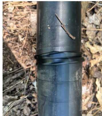
In this series of photos Boyd Butler and Jesse Brookings set the tee into clamp to fuse to the next section of pipe. They use a metal paddle run by the generator to heat the plastic on both sides and then clamp it together when hot to fuse the seams together
