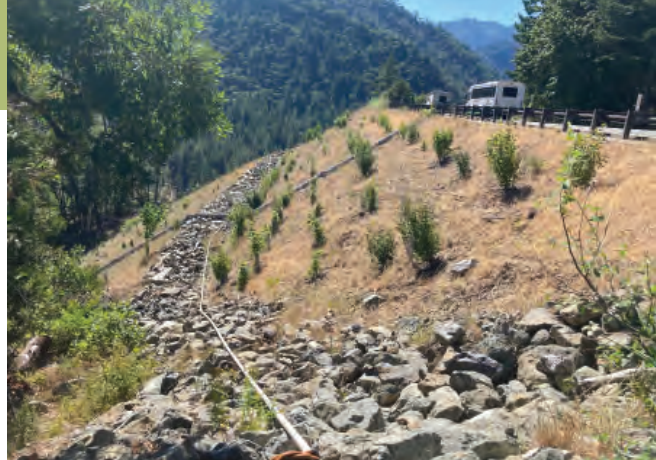
TCRCD plantings on the Collins Bar Curve Improvement Project
