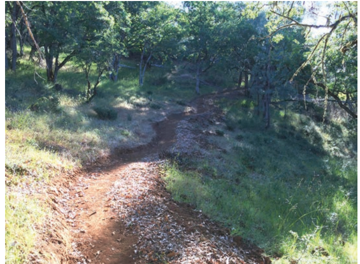
Trail maintenance on Jackass Ridge
