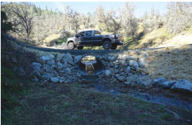
Culvert outlets looking downstream after repair.
