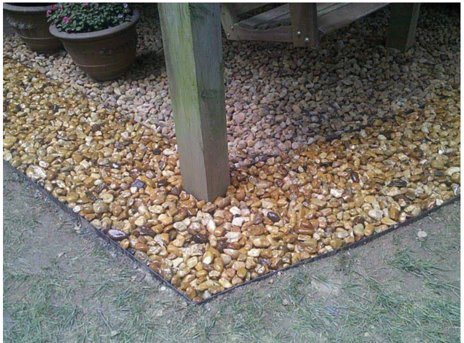
Gravel placed under the drip line around decks can help slow water and will increase infiltration.
