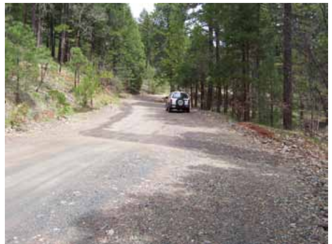
Rolling dips are designed to catch runoff and direct it away from the road surface into a carefully selected location.
