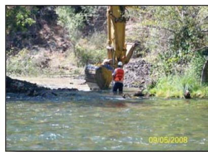
Constructing a side channel.
