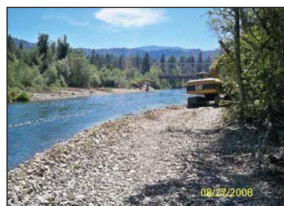
Constructing gravel bars near Lewiston.
